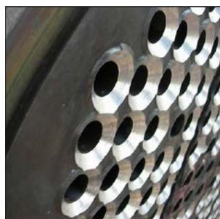
Completed strength weld removal.
